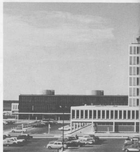
Administration building with air traffic control tower rises over approach road at Edmonton.
