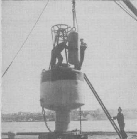
Replacing acetylene cylinder in buoy.
