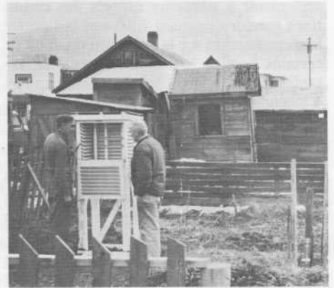
Voluntary Observer Harvey Howard (left) of Lumby, B.C. shows a friend the instruments in the Stevenson screen on his property.
