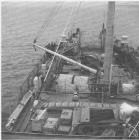
LIGHTING UP AN ISLAND —Photo far left shows East Ironbound Island as seen from the air. Left, CCGS Mink proceeds toward the island as crew lays the cable. Lower left, Sid Forward, base electrician, prepares a splice in the 7,200-volt cable. Fourth photo shows the 100-year old lighthouse, the ubiquitous hydro pole behind it signifying the last step in connecting the station to mainland electricity.
