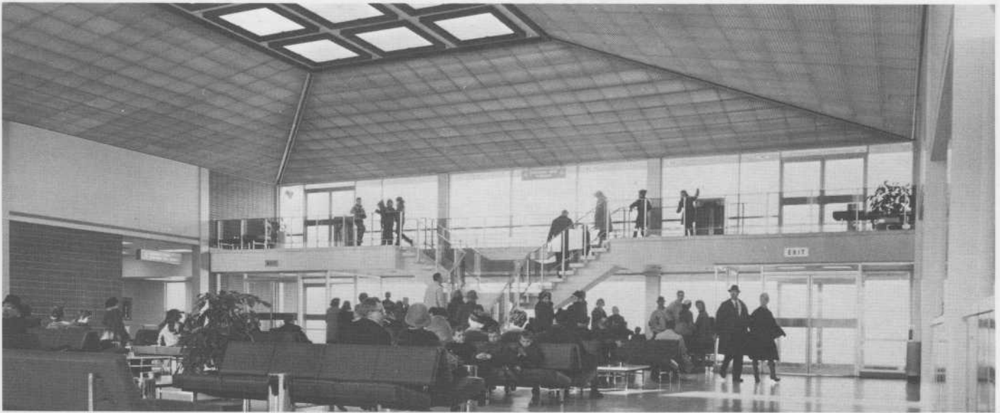
The spacious waiting area and the mezzanine overlooking the aircraft ramp at London Airport.
