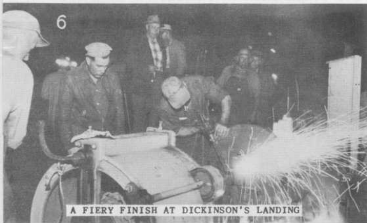
J.V. KELLY CUTS CONCRETE WITH OXYGEN LANCE
