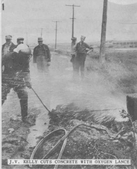
CORNWALL CANAL CREW RAZES WEIR AT LOCK 20 P. TROTTER, WELDER A. SAVARD, AND C. EYER
