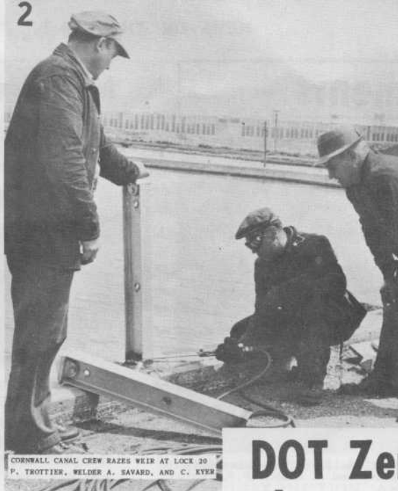
J.V. KELLY CUTS CONCRETE WITH OXYGEN LANCE
